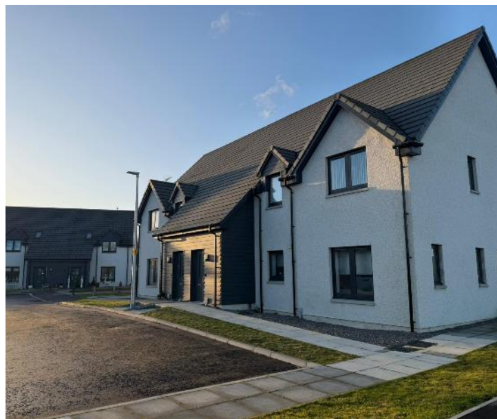
Affordable Homes at Beaully
